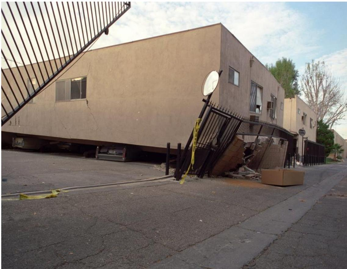
**Figure: Soft story of failure (Khan and Rawat 2016)**
